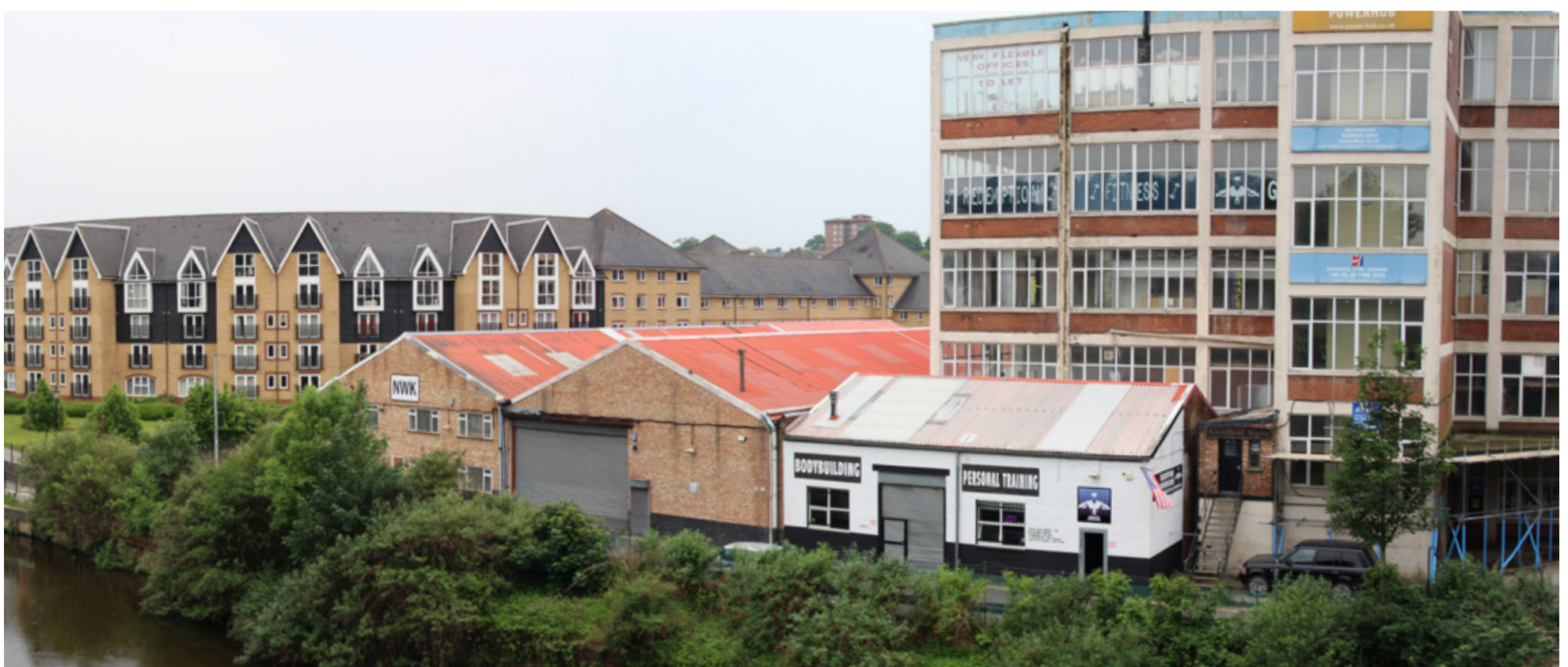
Powerhub site with Scotney Gardens beyond, seen from pedestrian footbridge over River Medway
